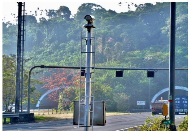
Formosa freeway Chiayi tunnel, Taiwan
