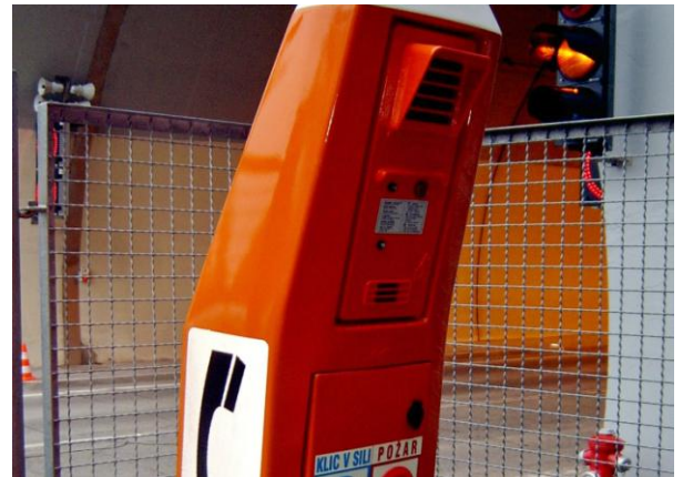
Ljubel tunnel, AUT/SLO, portal SOS
