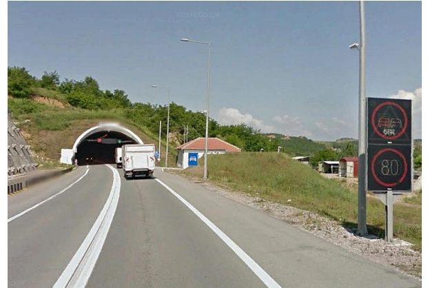
Straževica tunnel, SRB
