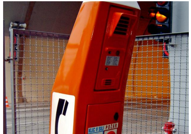
Ljubel tunnel, AUT/SLO, portal SOS
